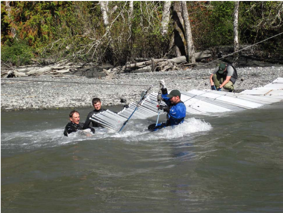
Figure 6. High river flows on August 7, 2013 made installation more challenging and operations more difficult (personnel safety was a major concern).
